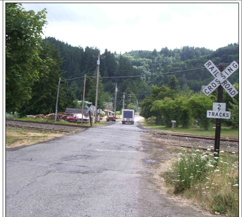
US-30 / OLD MILL TOWN ROAD COLUMBIA RIVER RAIL CROSSING WESTPORT, OREGON
